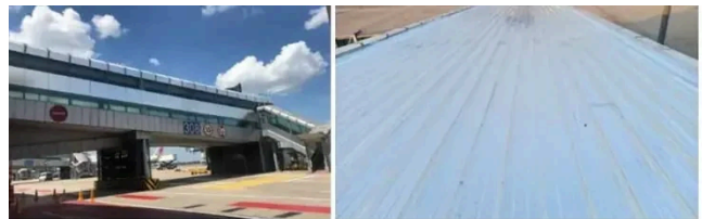
Post construction appearance photos
